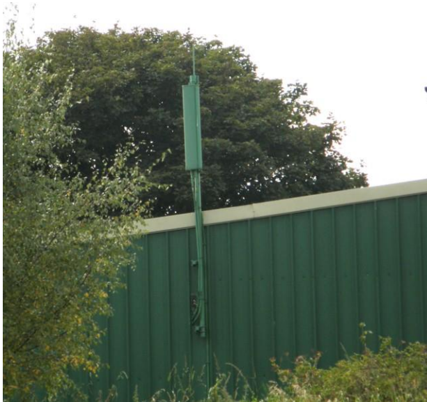
Transmitter Site Photo
